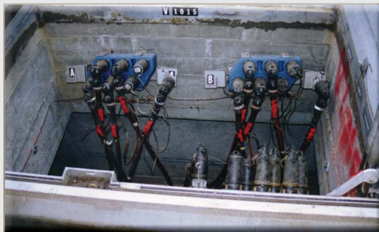
Manufactured to ANSI/IEEE Standard 386 Vault Installation using 6 Point Stacked Style Junction Bars
